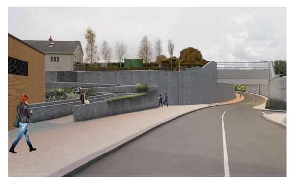
IÉ are proposing to lower both the road and pedestrian and cycling facility to the same level. This is entirely unnecessary and is against best practice across Europe. The pedestrian and cycling facilities need only be lowered as required since they do not require such a large clearance as trucks and buses on the road. This avoids creating a large unnecessary hill for pedestrians and cyclists at the underpass.
